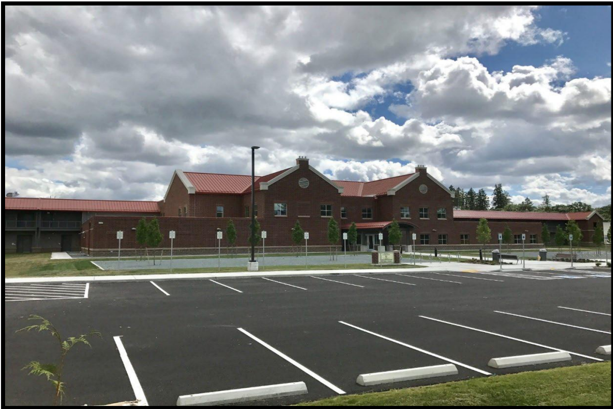
International Operations Readiness Center (IORC) – Joint Base Lewis McChord, WA
